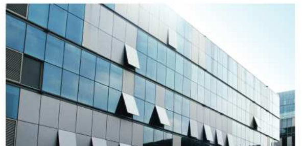
Exterior Wall Construction (Chameleon)
