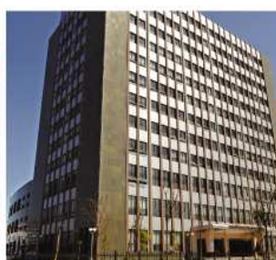
Exterior Curtain Wall Construction(granite)
